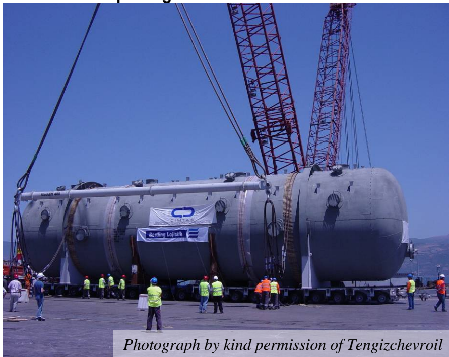
Photo 2: Transporting a 7.5m diameter x 29m t-t Claus Reactor (286 tonnes)
